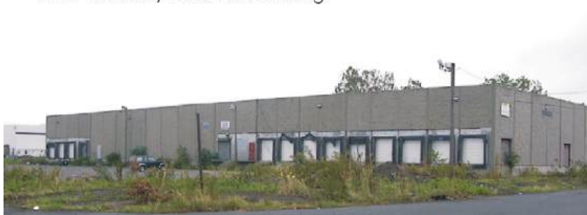
Making a real estate purchase takes a lot of legwork – I looked at 46 buildings and 23 pieces of land before I fell in love with this site in Jersey City
