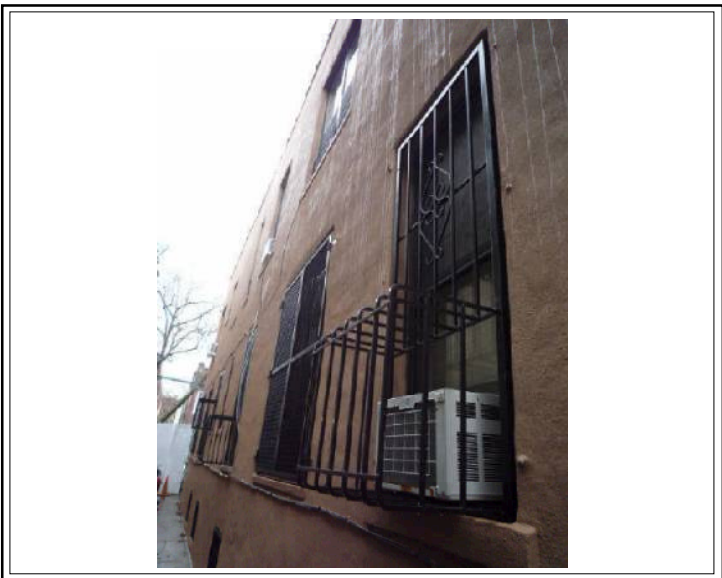
Steel Bars without Latches- Unit 1 bedroom 2 Subject to removal or installation of latches
